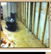
however the cost involved in correcting that cheaper system can be astronomical. Out of all the mistakes made potentially the worst is not floating concrete under the stud walls. This promotes mold and water intrusion behind the wall and WILL have to be replaced. Here is a picture of a cheaper system left uncorrected.
