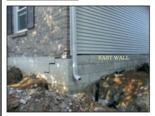
Perma Jack system installed to correct - 3 3/4" settlement in North/East corner of structure. East wall had rotated out 1 1/4" and corrected to 1/4" without causing additional damage to structure. Settlement on North wall was corrected to 34" Lift was stopped to prevent additional damage if grade beam was carried back to original elevation. Structure was stabilized and aesthetic repairs were made.
